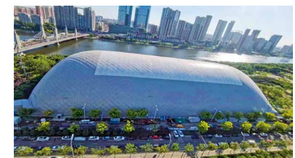
Fully-enclosed Construction in Foundation Pits with Air-supported Membrane Dome
