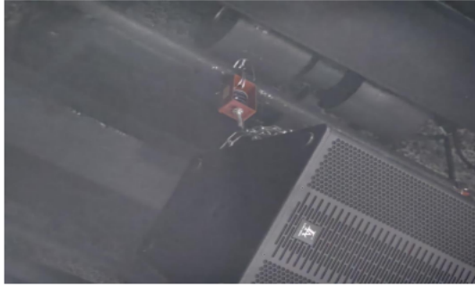
场内音响加装减震弹簧
